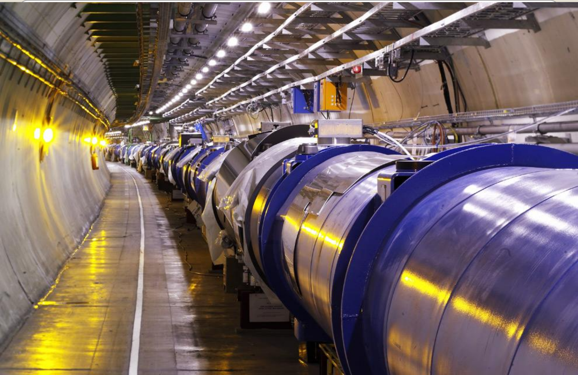
View of the LHC cryo-magnet inside the tunnel. (Maximilien Brice, © CERN)
